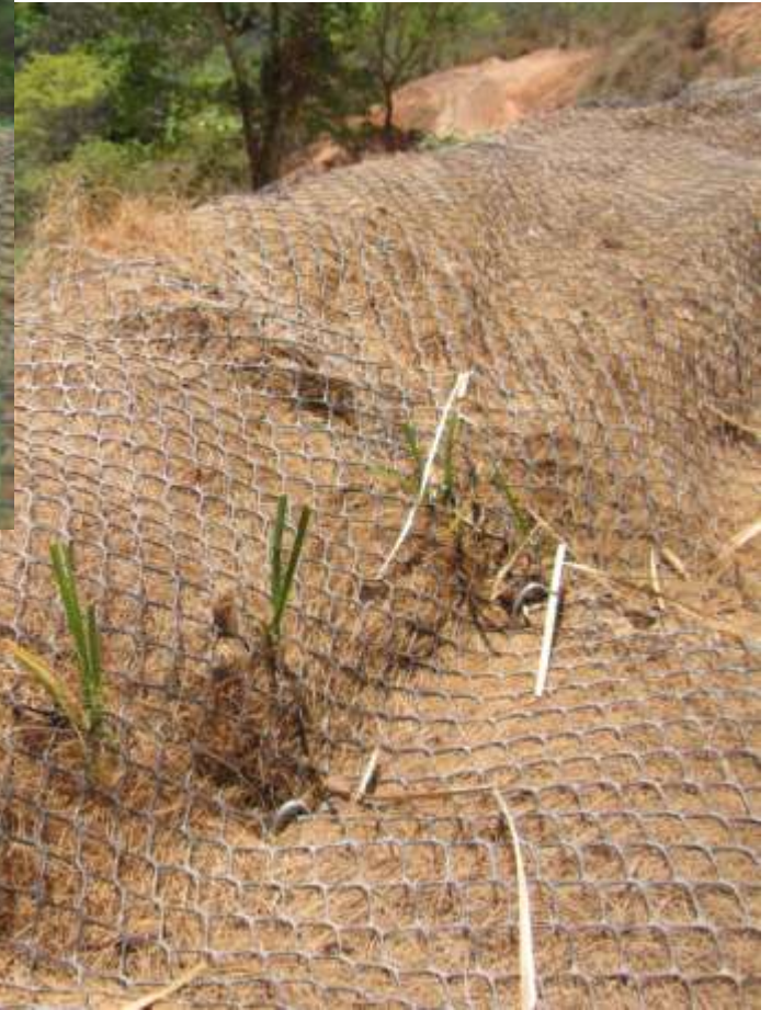
Vetiver emerges through coconut blanket
