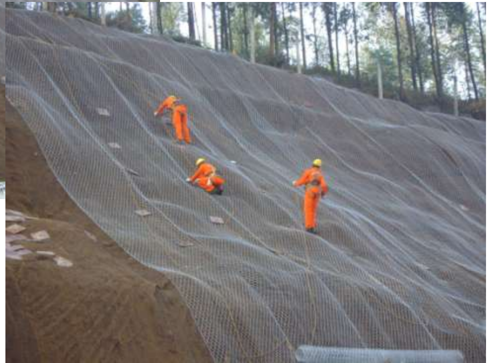
Wire mesh laying for extra structural protection
