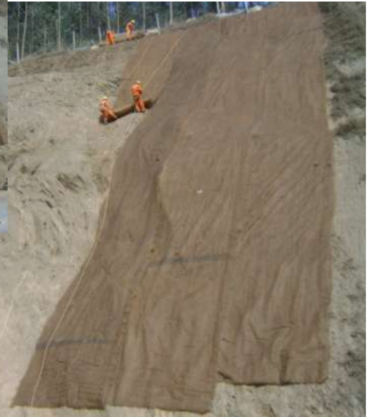
Coconut blanket laying
