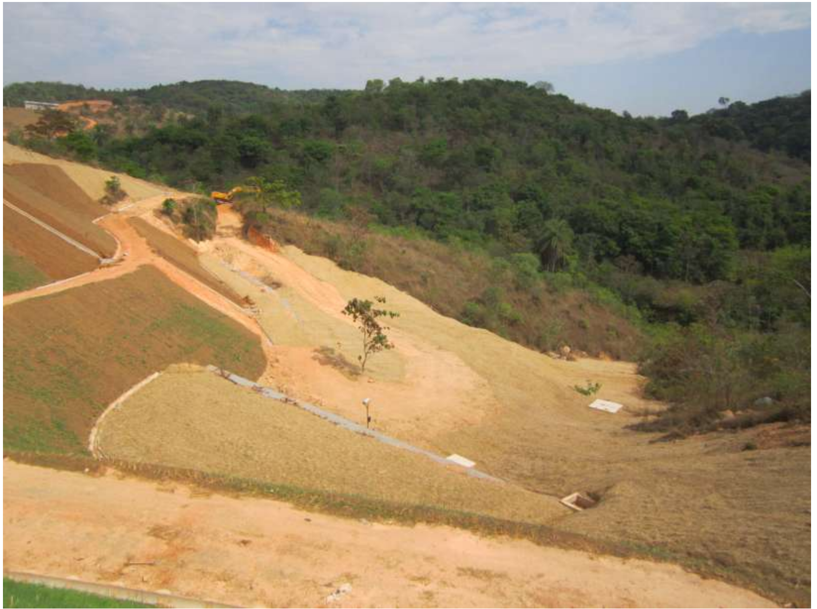
Another examples of very complex set of cut and fill slopes
