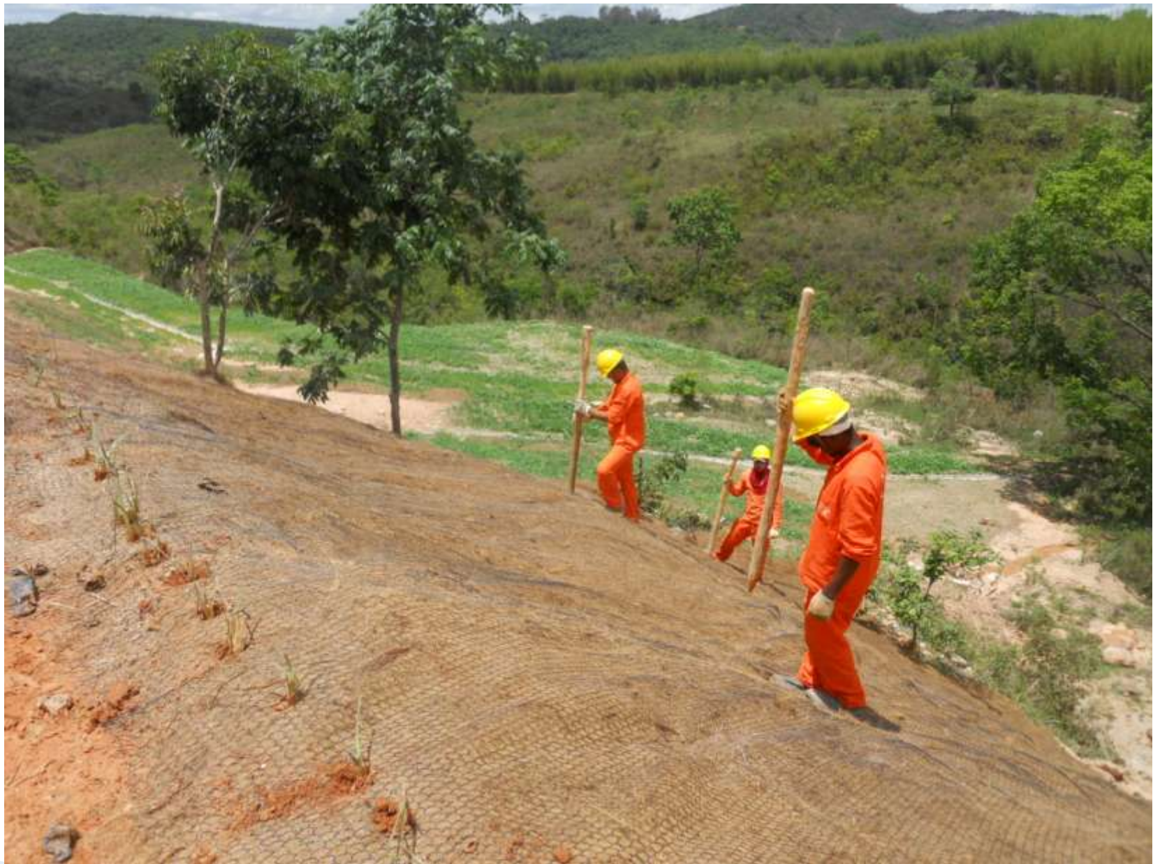
Using sharp poles to pierce coconut blanket for planting
