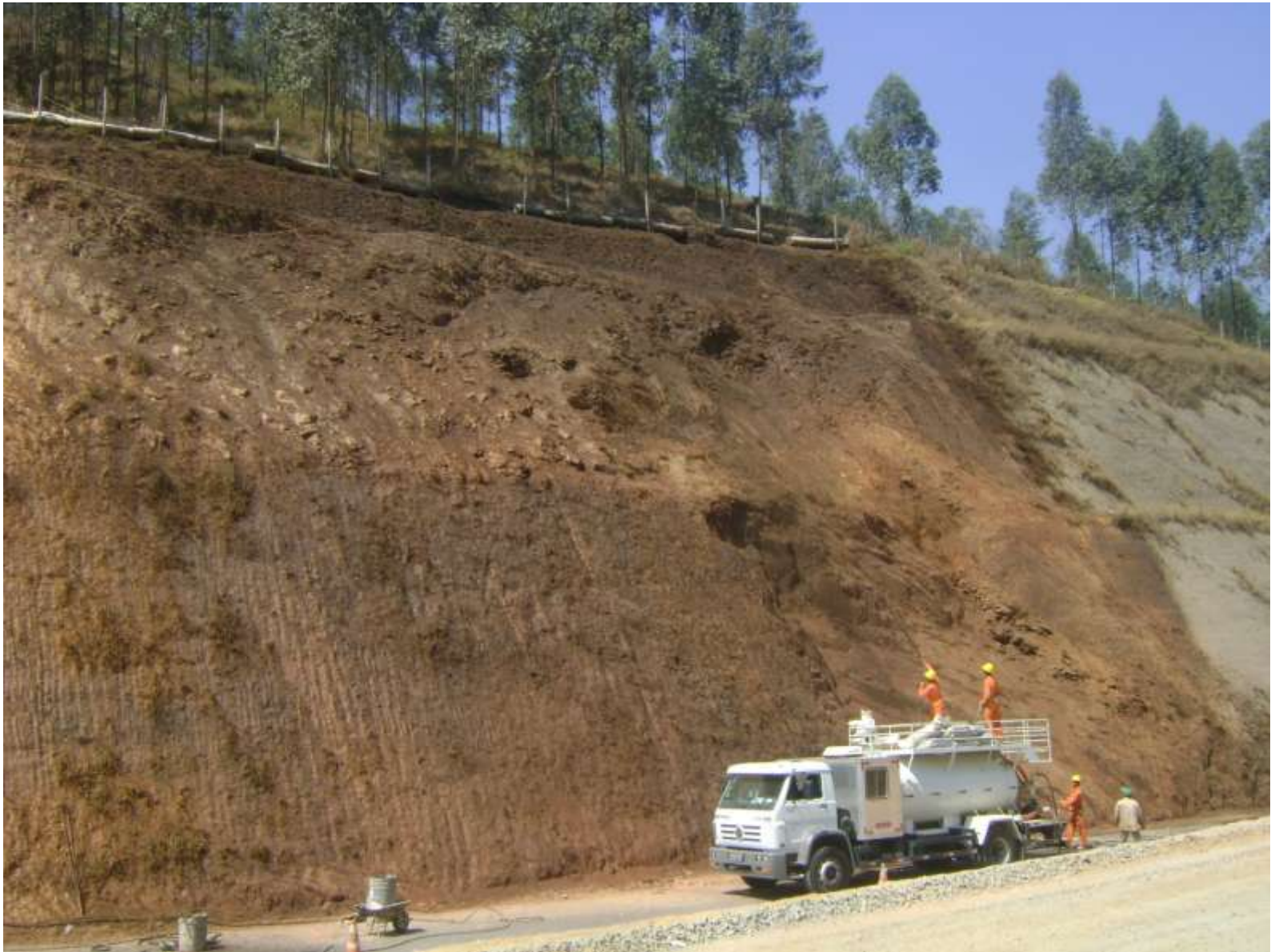
Hydroseeding after minimal surface repair
