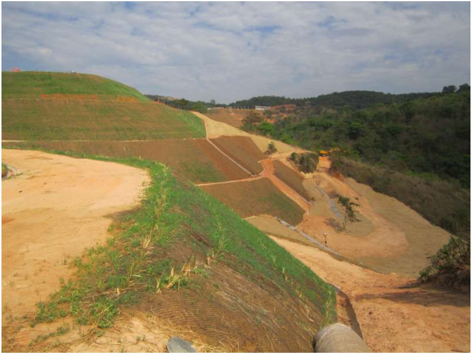
A highly complex set of cut and fill slopes
