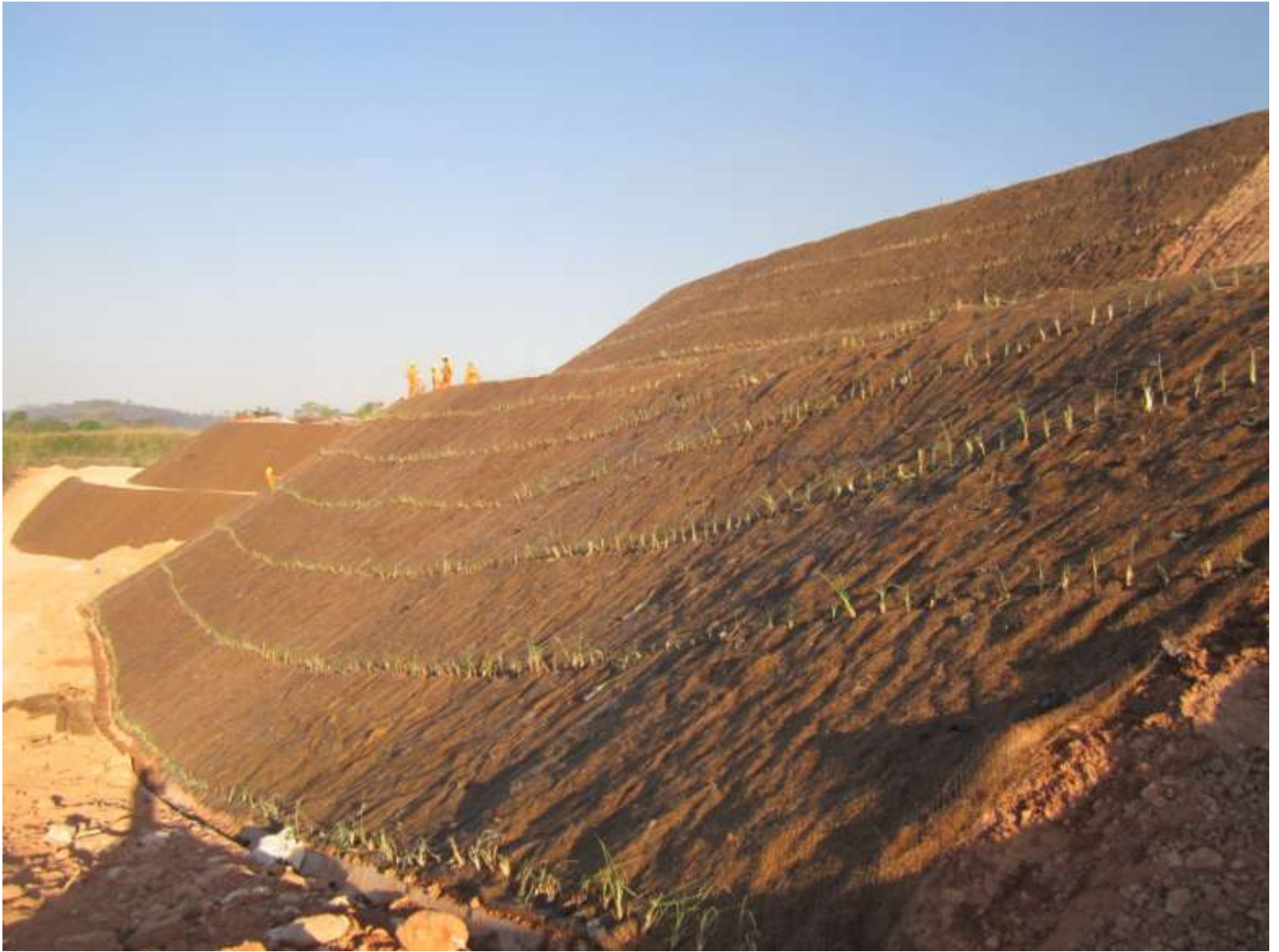
Vetiver planting on contour line on slope protected with coconut blanket
