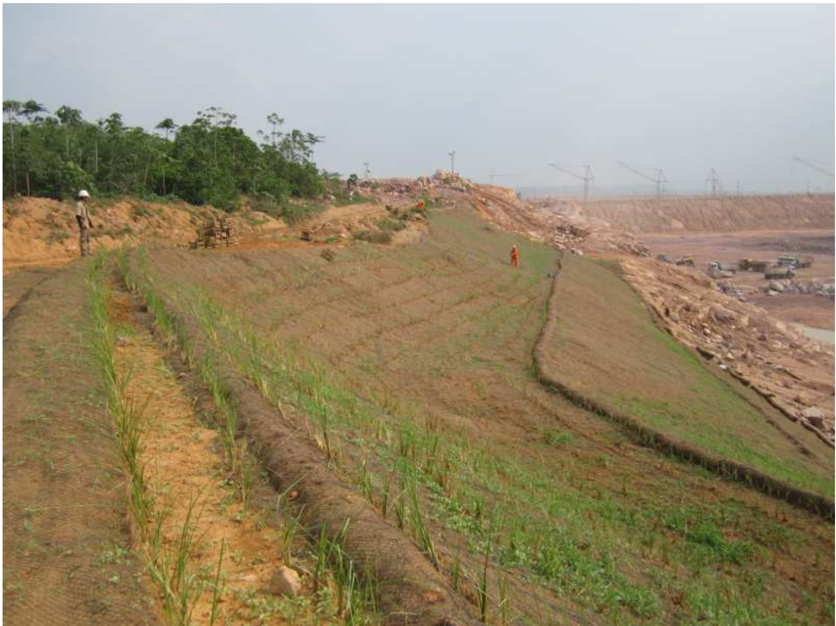
Vetiver planting on combination of coconut blanket and Bermalonga, (a Deflor product made from straw and coconut fiber) on highly erodible sites
